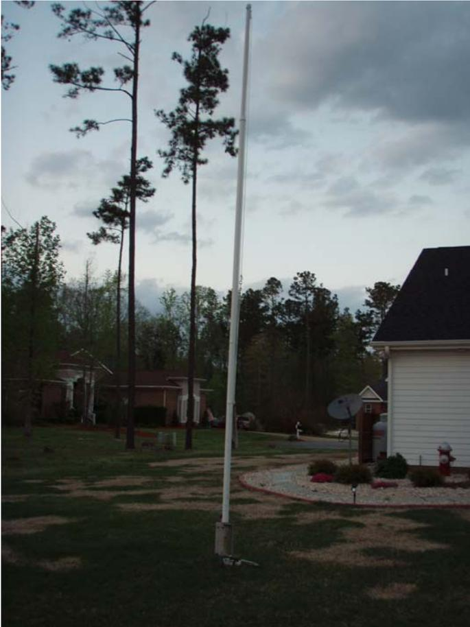
It's a Hustler 5-BTV Vertical (minus the 80M resonator) mounted on a DX Engineering Tilt base which, in turn, is bolted to a 1 3/4" pipe driven into the ground. The ground system consists of 2 quarter wavelength radials for each band (#14 solid wire buried about 1" in the ground). The antenna is covered with 2" and 1 1/2" PVC tubing.
